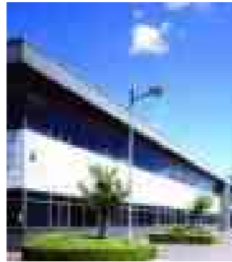
Redhill Data Centre. Redhill, Great Britain.
